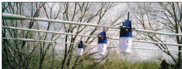
Wireless AutoRANGER Fault Indicator installation.
